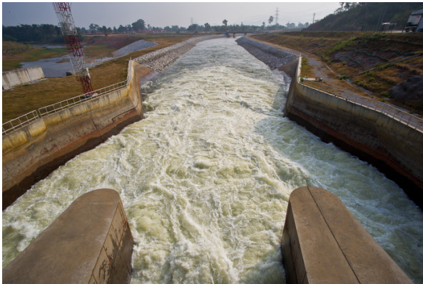
A reservoir of the Nam Theun 2 Dam.
