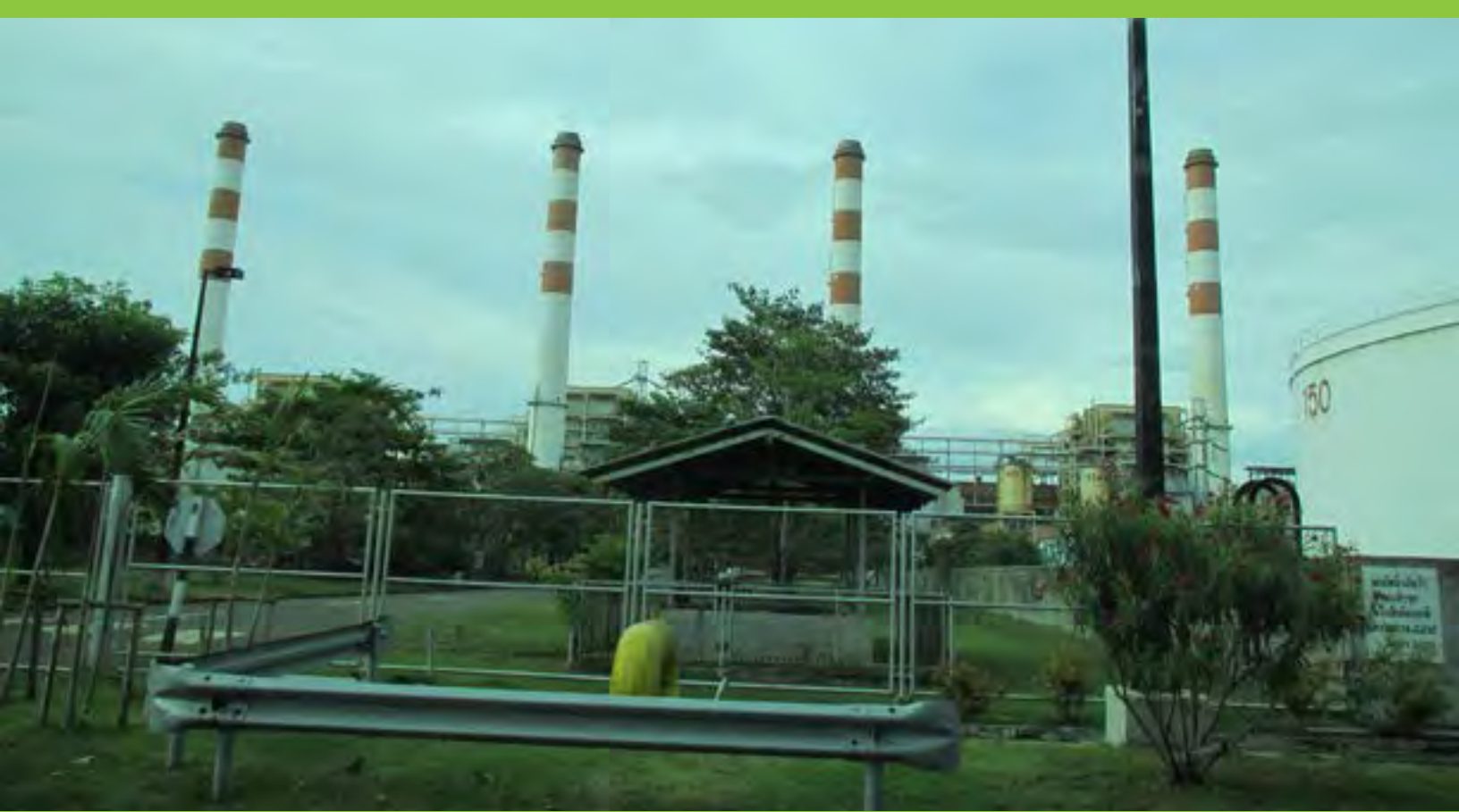
1375 MW Ban Pakong combined cycle gas turbine power station, Thailand
