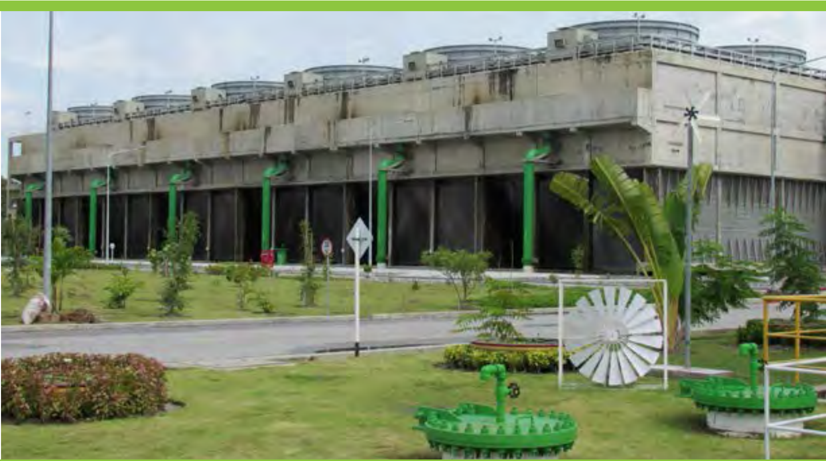
Water cooling at Bang Pakong combined cycle gas turbine power station, Thailand
