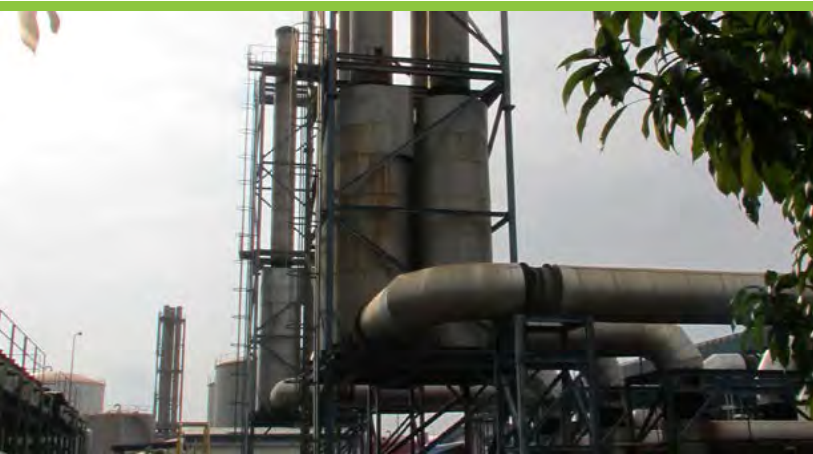
10 MW oil-fired power station, Phnom Penh
